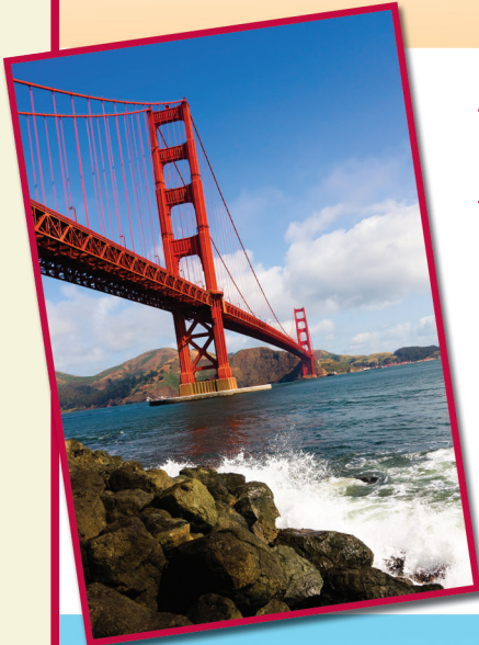
After four years of construction the opening celebration of the Golden Gate Bridge was May 27, 1937. Many said it couldn't be built. It is considered one of the Wonders of the Modern World.
